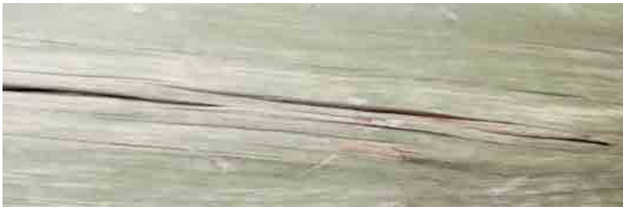
Long splits from the centre right to the base; sign of decaying and rot.
